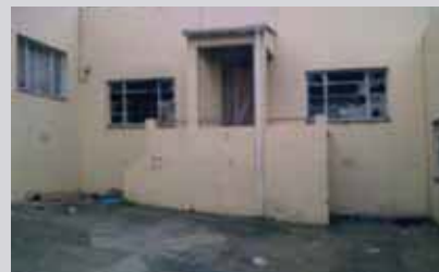
Santos complex before the upgrade.
